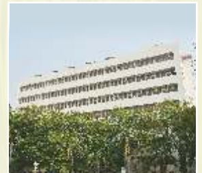
Central Library Block-C
